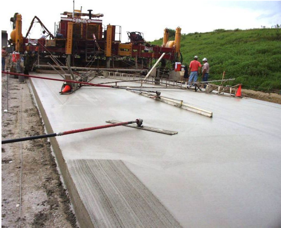
Hand float and straight edge
