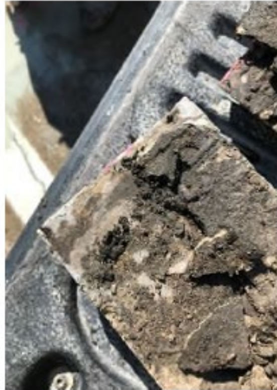
Packed slurry below backer rod.
