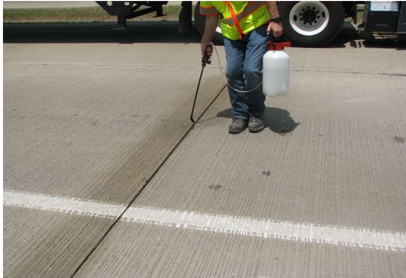
Application of a penetrating sealer to concrete
