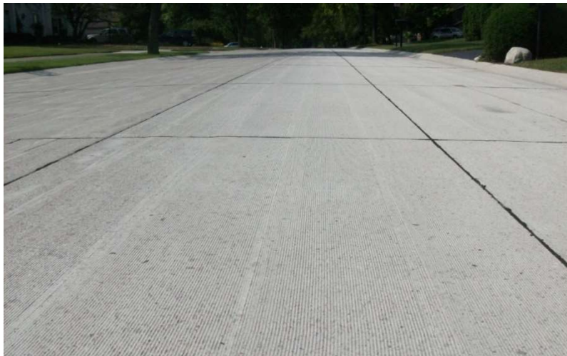
Example of a diamond-ground street
