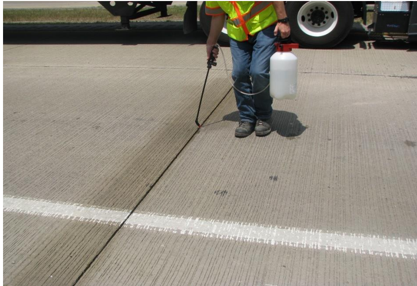
Application of a penetrating sealer to concrete
