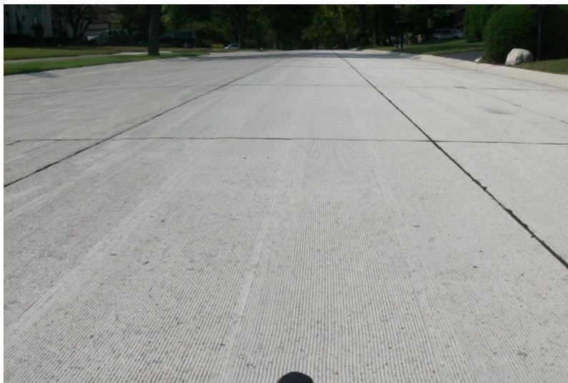
Example of a diamond-ground street
