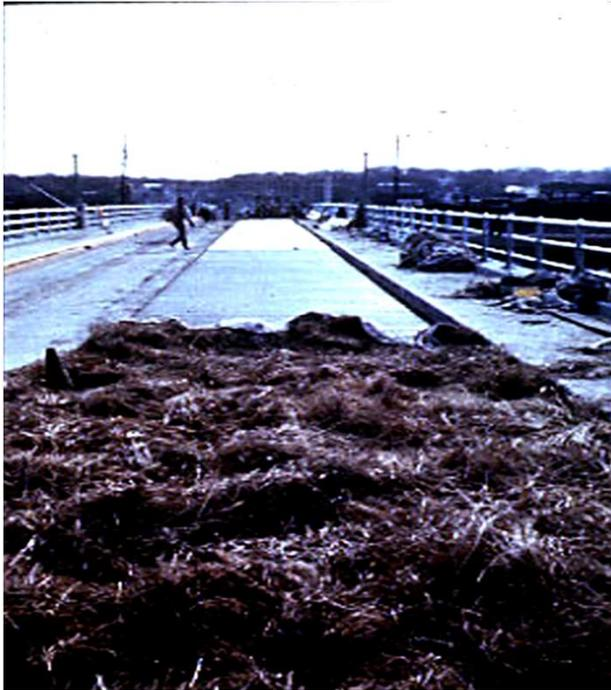
A minimum of 1 ft. is required to provide the necessary insulating (R) value. Straw or hay must be covered with visqueen (poly) to securely hold it in place.
