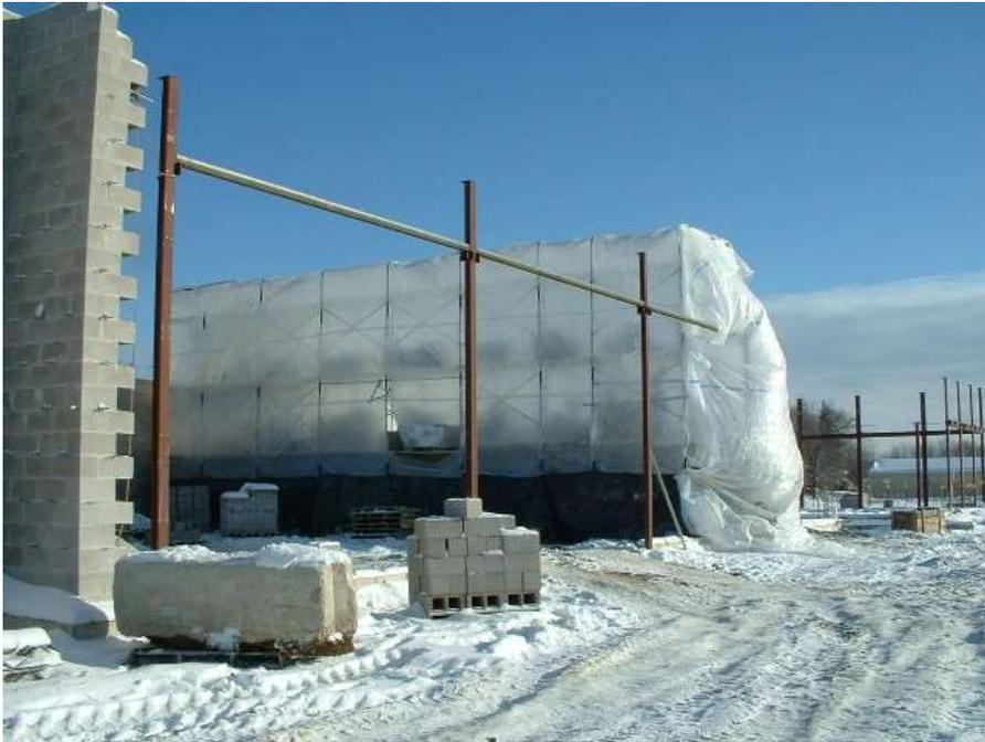
Heated enclosures are expensive to construct and operate but allows for construction to continue during cold weather conditions.
