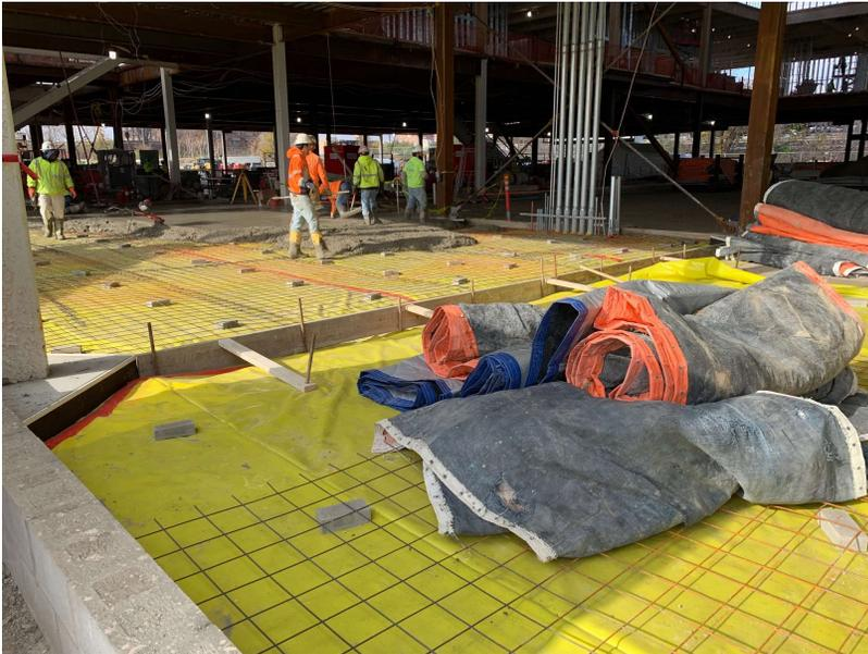
Provided that necessary precautions have been taken, concrete can be placed year round. Such precautions for cold weather construction include:
