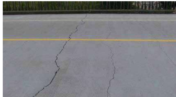
Transverse Cracking
