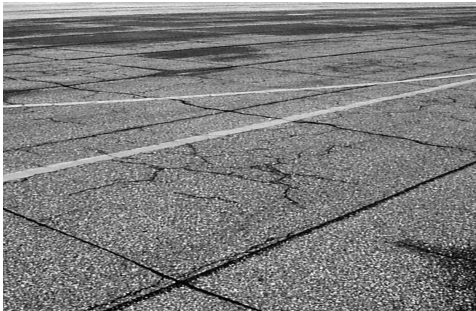
Reflective Cracking
