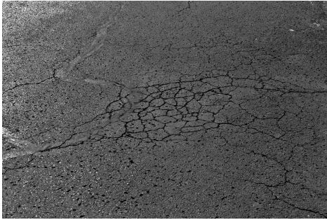
Alligator Cracking
