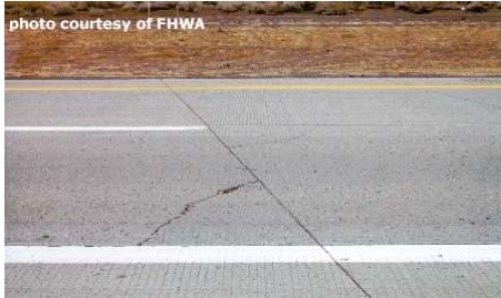
Corner Cracking
