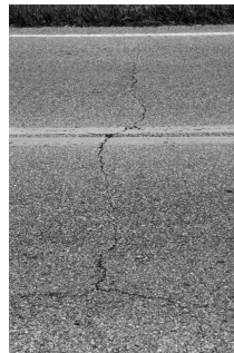
Transverse Cracking
