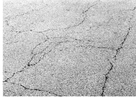
Block Cracking
