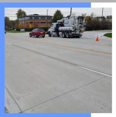
Construction on this stretch of Lahser Road in the City of Southfield started July 26, 2017 with a total road closure on the south end of the roadway between Civic Center Drive and eastbound Northwestern Highway service drive. This allowed Florence Cement crews to replace all of the existing pavement with a smooth-riding, 10-inch-thick plain concrete pavement with skewed transverse joints.
