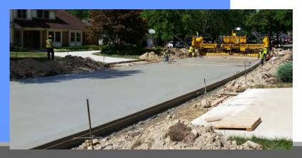
The original concrete pavement in Independence Commons was constructed in 1967, and after close to 50 years of service, required significant rehabilitation. Several options were considered by the city of Farmington Hills including an alternate bid for full depth concrete or asphalt replacement. In the end, full concrete replacement was chosen.
