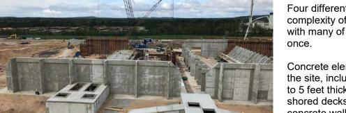
Four different forming systems were used due to the complexity of the formwork and scheduling of the pours, with many of them custom built and some used only once
