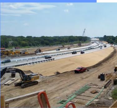
After nearly 20 years of planning, Segment 1 of the I-75 Corridor Modernization was bid in June 2016 as a Design-Build, Alternate Bid project. MDOT short-listed three bidders for the project, and of those short-listed, all three utilized concrete pavement. Asphalt was only used as a temporary pavement.
