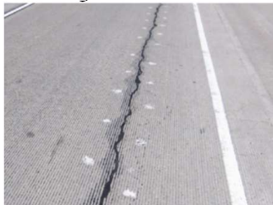
b. Cross-stitched longitudinal crack
