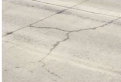
Wheel path cracking-debond & fatigue cracking of overlay
