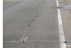
Reflective crack-not cutting a joint over existing crack
