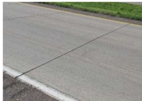
Mid-panel cracking
