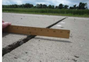
Transverse joint faulting
