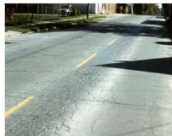
Wheel path cracking-debond & fatigue cracking of overlay
