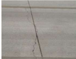
Late sawing/or not sawing over existing joint/crack
