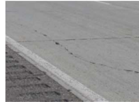
Cracking due to misaligned dowels
