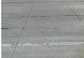
Transverse reflective cracking
