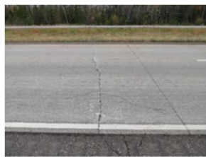
Transverse reflective cracking
