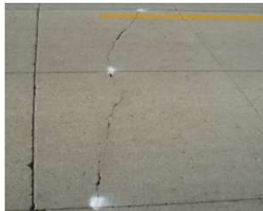
Mid-panel cracking
