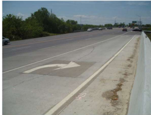
Figure 6.7 Longitudinal cracking due to longitudinally bounded variation in pavement support
