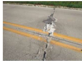
Longitudinal cracking in wheel path
