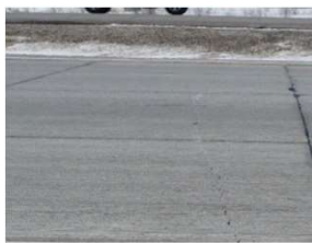
Mid-panel cracking
