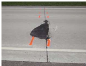
Cracking- misaligned dowels
