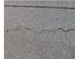
Reflective crack-not cutting a joint over existing crack
