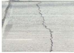
Late sawing/or not sawing over existing joint/crack
