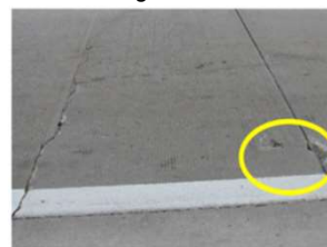
Cracking due to misaligned dowels
