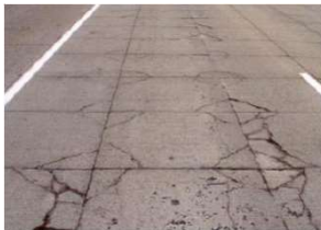
Transverse joint faulting
