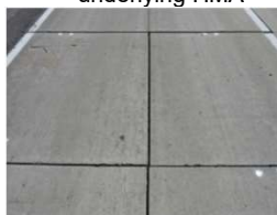
Mid-panel cracking
