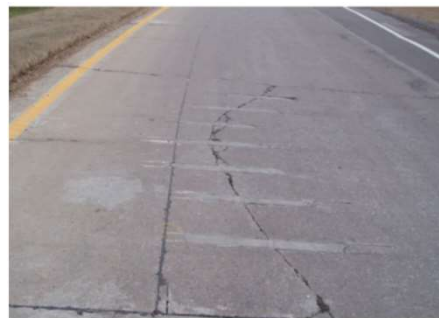
b. Slot-stitched longitudinal crack
