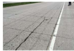
Longitudinal cracking in wheel path
