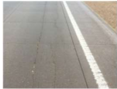
Cracking- misaligned dowels
